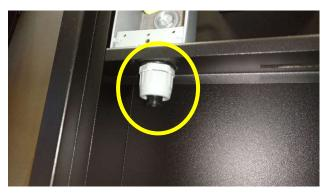
Figure 8 - Lower Nipple for AC Electrical Connection
