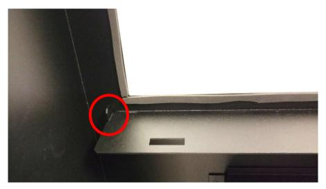
Figure 14 - Detail of Alignment Angle Stop
