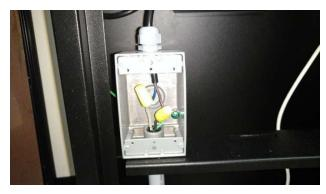
Figure 10 - Connect Incoming AC Power per local code and NEC
