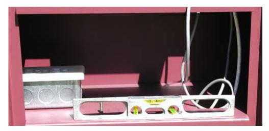
Figure 6 - Ensure Post is Level
