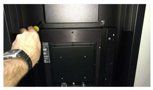
Figure 18 - Tighten #10 Nuts with 3/8" Driver
