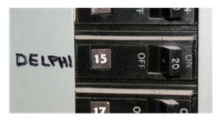
Figure 12 - Examples of Properly Labeled Circuit Breaker
