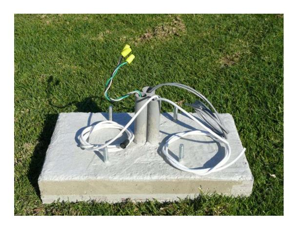
Figure 2 - Completed Footing
